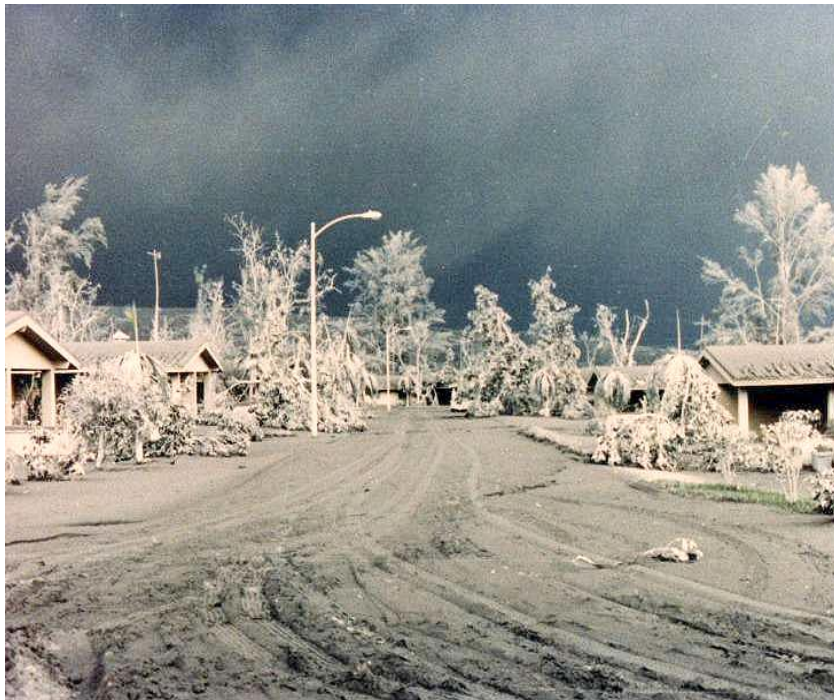
Figure 6: Base housing at Clark AB covered with ash after the eruption. Many buildings' roofs collapsed under the weight of the ash.
