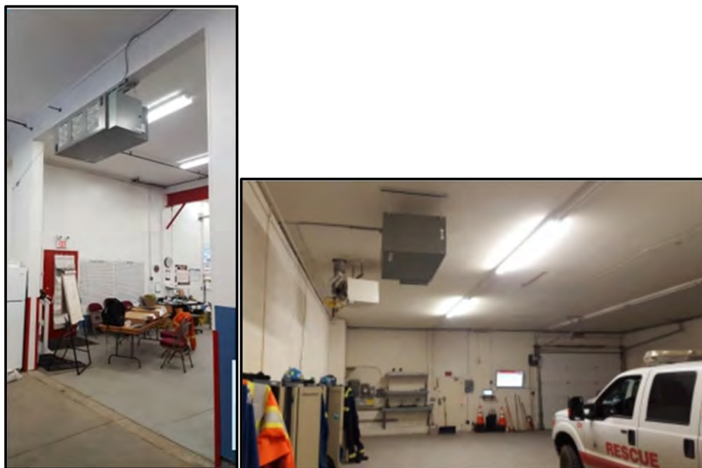
Exhibit 5-2 Photos of Ceiling-mounted Amaircare ES3X Tri-Carbon Heavy Duty Air Filtration Systems for Heavy VOCs
