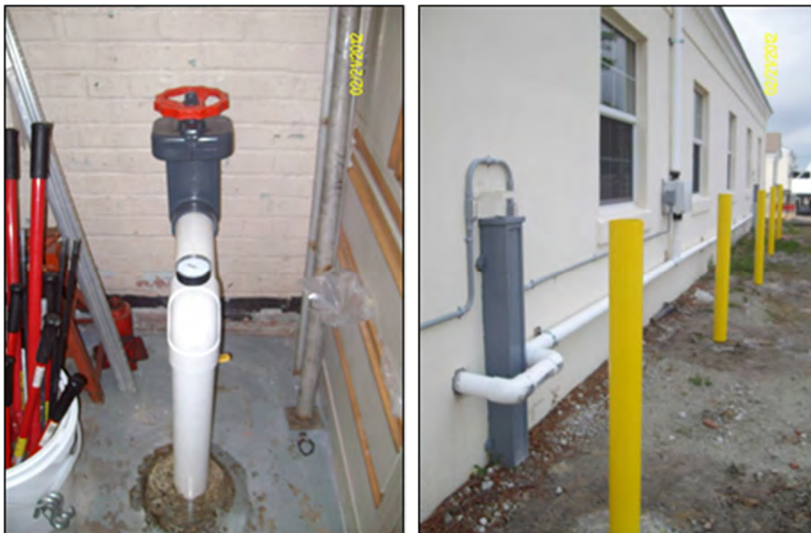
Exhibit 5-1 Example of SSD Piping at a U.S. Department of Defense Facility
