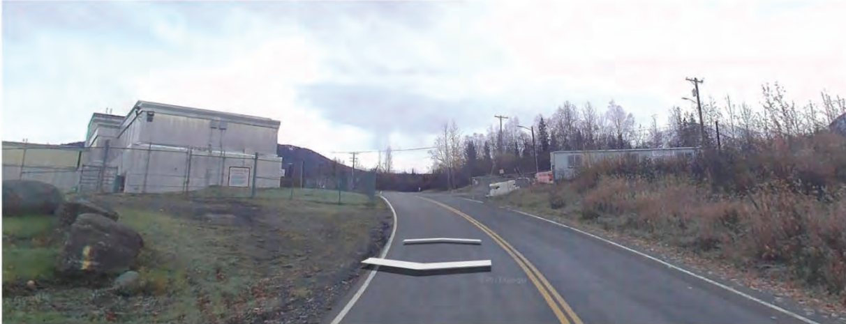
Figure 5. Looking east at Arctic Valley Road and the existing water treatment plant.
