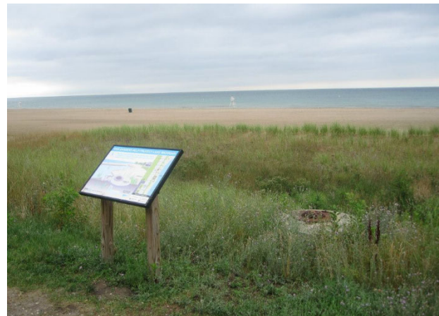
Dry Infiltration basin at stormwater outfall to capture and treat stormwater prior to public beach; provides co-benefits of aesthetics, buffer to water body, and habitat.
