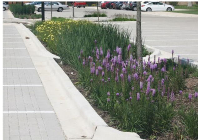
Parking lot with bioinfiltration swale, curb cut, and permeable pavers.
