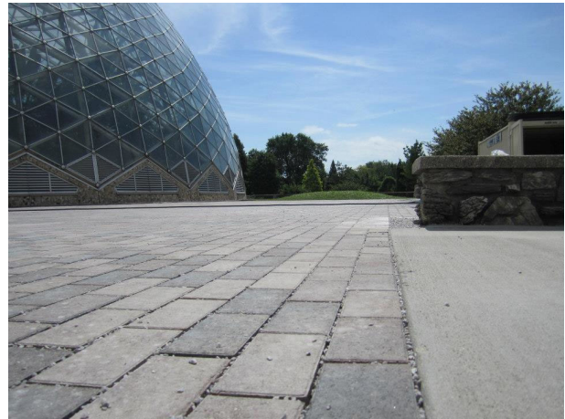
Rainwater is collected into an underground cistern from roof downspouts overlaid with 10,000 sf of permeable pavers. The cistern is lined with an EPDM liner, filled with large wash stone and "GeoBlocks" to create a base and a large water holding capacity. The harvested rain water is re-used for watering landscaping and greenhouses.
