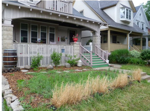
Residential example showing roof downspout disconnect to a rain barrel and a bioinfiltration basin; provides co-benefits of rainwater harvesting and green space; bioinfiltration can be landscaped with either turf or native plants.
