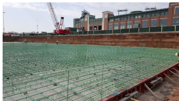
The start of a 270,000 cubic foot underground concrete vault to serve as an underground stormwater basin in a development with limited space.
