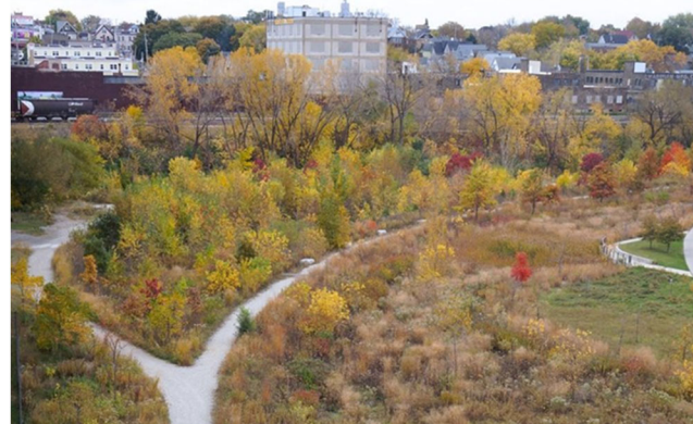
A series of constructed wetlands adjacent to a river that collect and treat stormwater from a light industrial 100-acre development with co-benefits of providing green space for a park and trail system, aesthetics, buffer to a river, and habitat.
