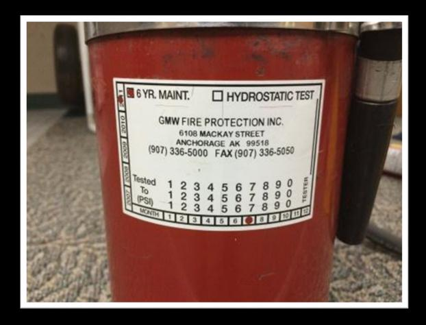
If there is a service collar present, you can use the Maintenance Label to calculate the last maintenance date (s). The label will list the last 6-year maintenance date or the last 12-Year hydrostatic test date.
