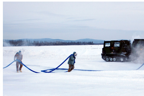
Soldiers from the 56th Engineer Company spread water to thicken a path of the Tanana River's frozen surface during an ice-bridge construction project. (U.S. Army photo/Staff Sgt. Matthew E. Winstead)
